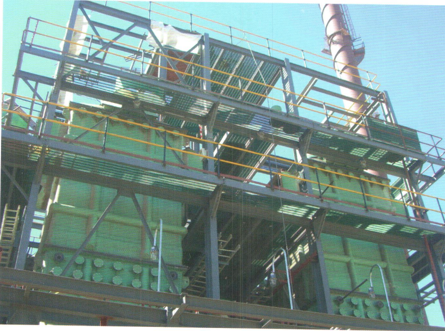
Hindustan Zinc Acid Plant, India: Beltran Wet ESPs virtually eliminate particulate re-entrainment, achieving 99.9% collection efficiency and faster throughput.
