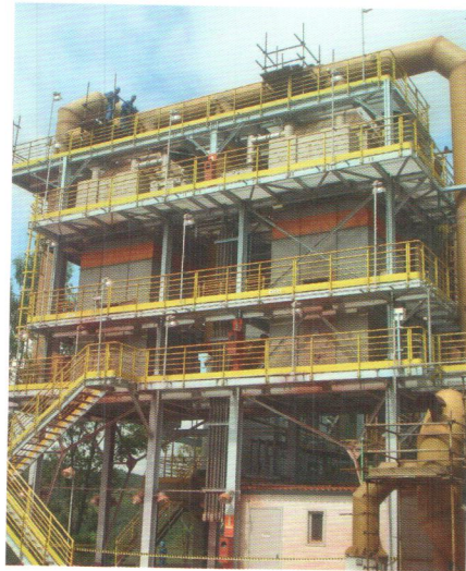
Anglo-Gold Ashanti, Brazil: Beltran WESPs effectively clean refinery gas of submicron-scale impurities, acid mists.
