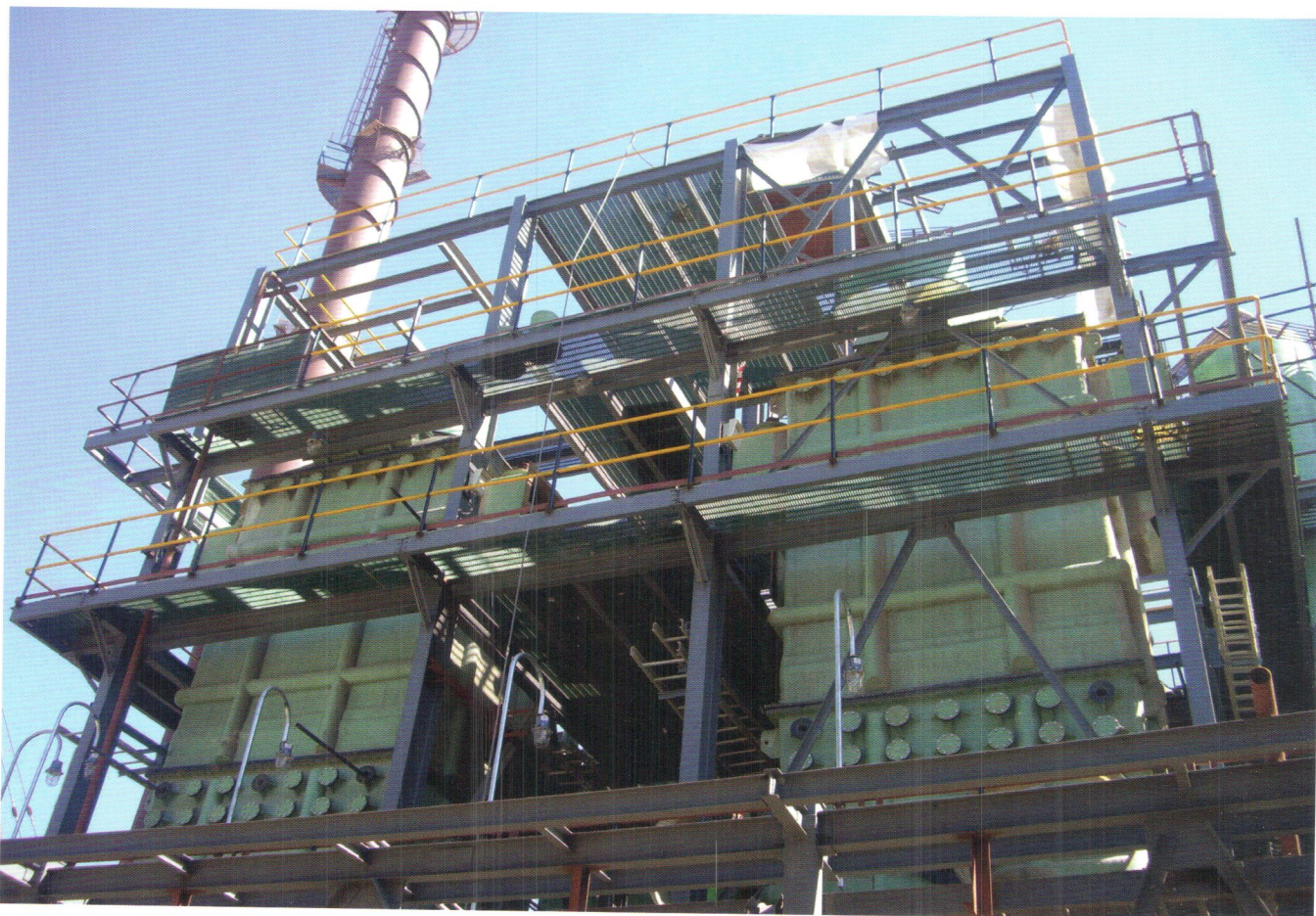
Hindustan Zinc, Udaipur, India uses Beltran WESPs to control submicron size particulate emissions from their smelter operations.
